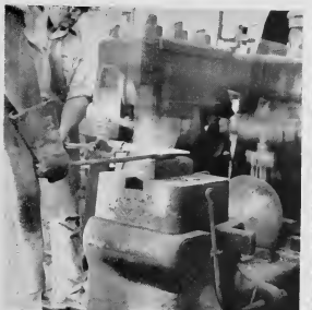
The days of the blacksmith shop under the spreading chestnut tree are gone, but sinewy hands are still needed in the Mechanical Department blacksmith shop (15). Here the camera catches the blurred stroke of a powerful mechanical hammer as it beats a piece of metal, glowing at white heat, into shape.
